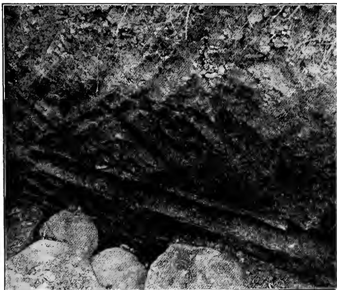
FIG. 77. Section of a 20-year-old tile drain in heavy clay soil. Note the more open structure above the drain.
